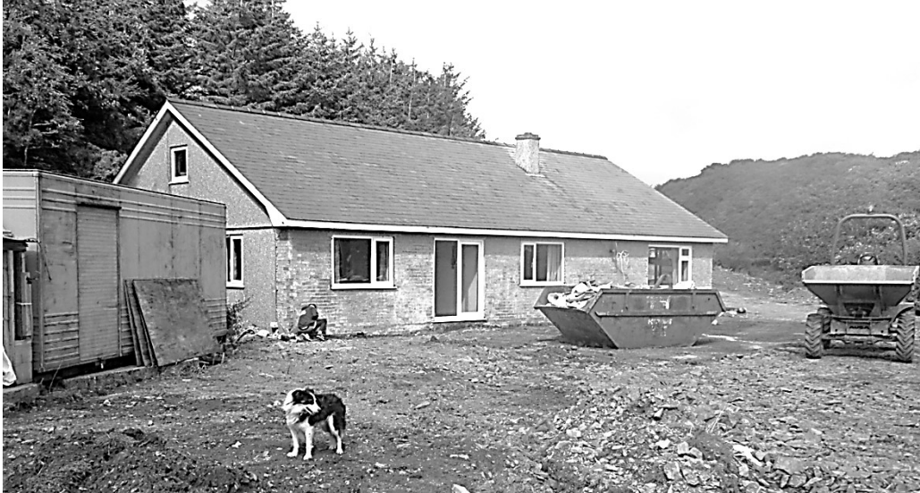
Figure 69: Bungalow where wiring installation is planned
